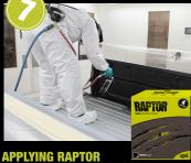
With the air pressure set at 60 PSI (4 Bar), apply two coats of RAPTOR allowing 45-60 minutes flash off between coats.
